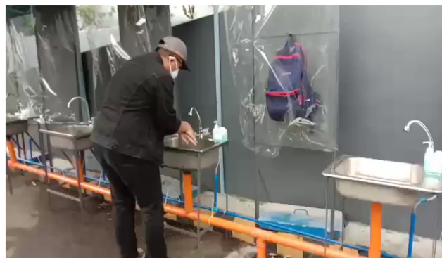
Figura 3. Bag hangers and handwash sinks in Sanitation Walkway
