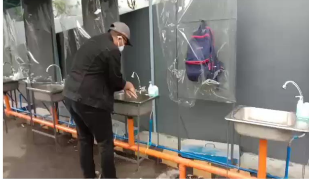
Figure 3. Bag hangers and handwash sinks in Sanitation Walkway
